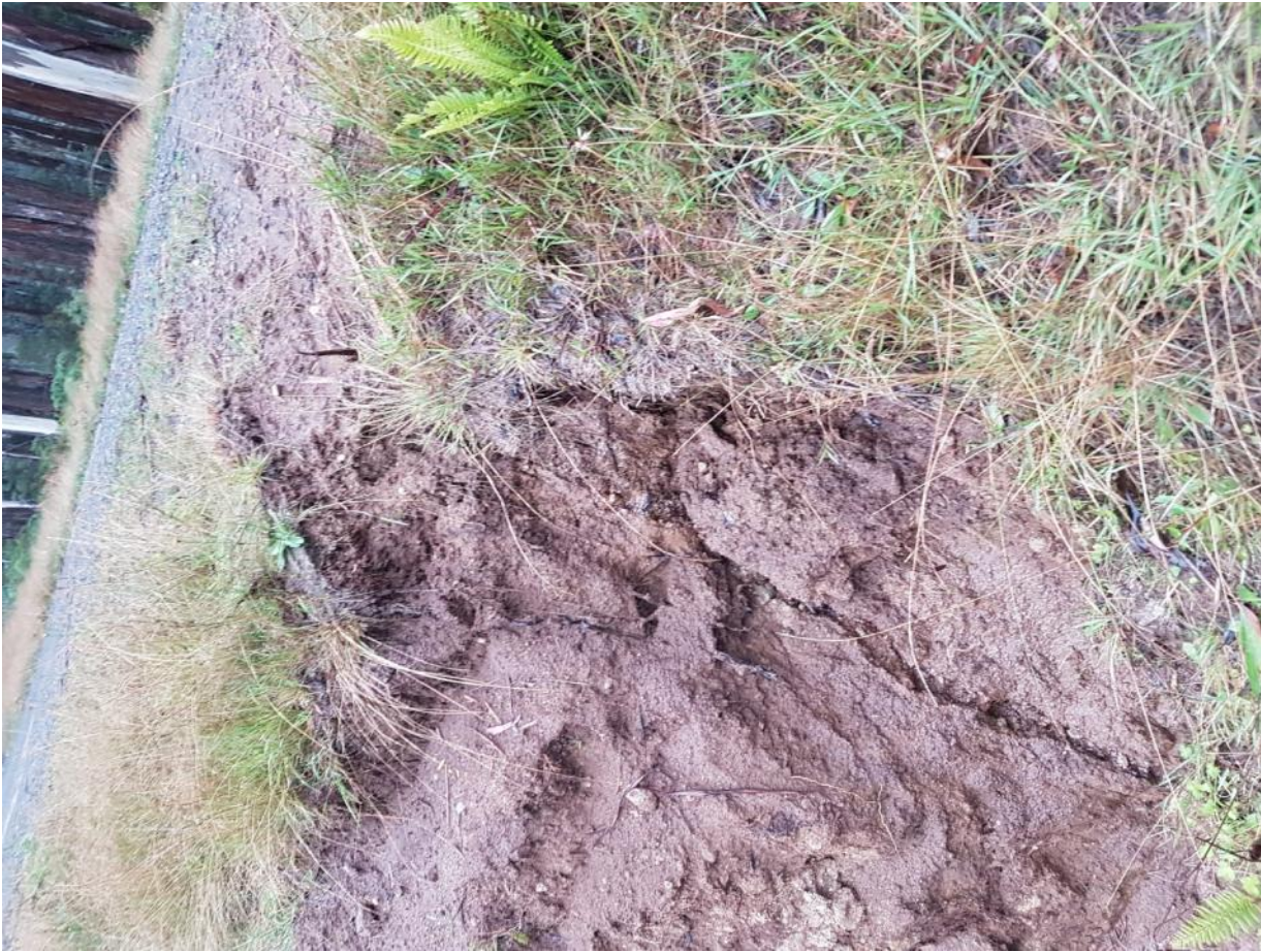
Overflowing silt trap on Snobs Creek Road south of Snobs Bridge adjacent to active coupe
