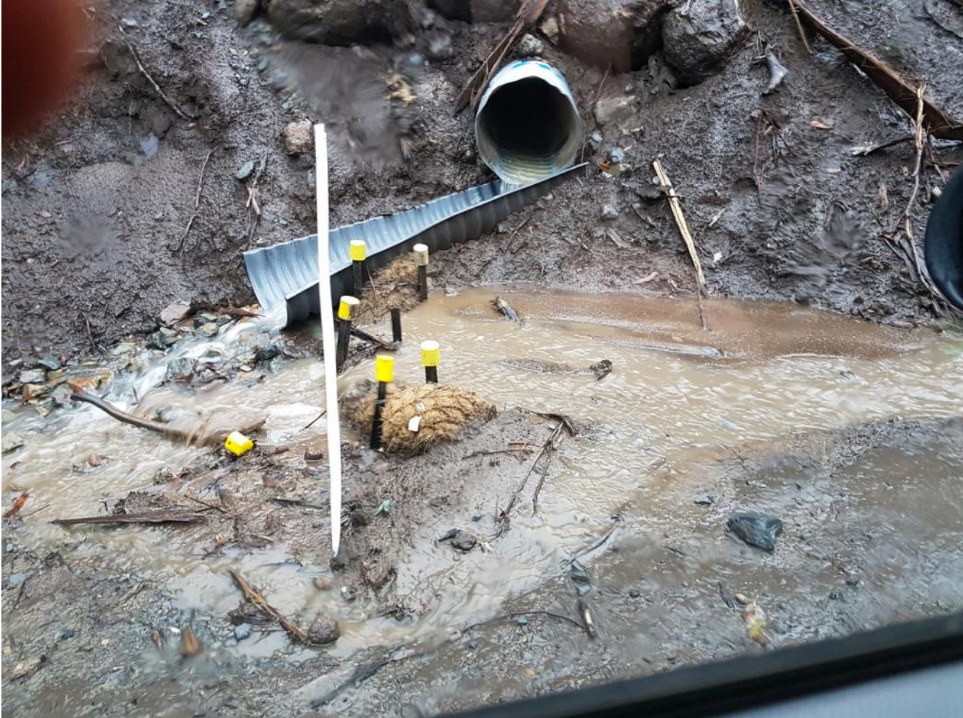
Overflowing silt trap on Snobs Creek Road south of Snobs Bridge adjacent to active coupe
