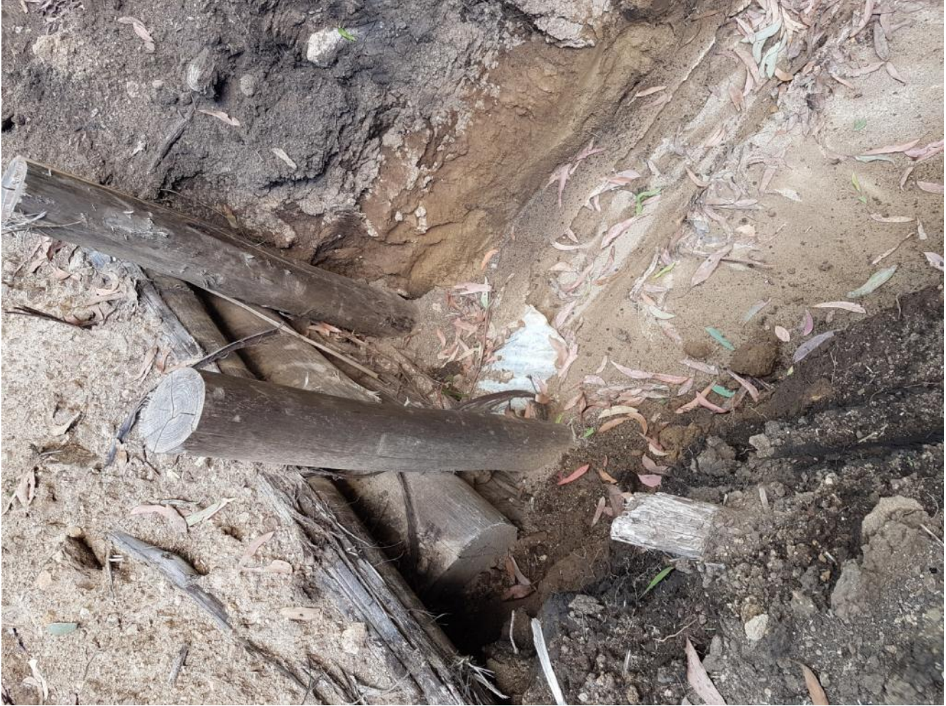
Another blocked culvert exit under Gnu access road (17/3)
